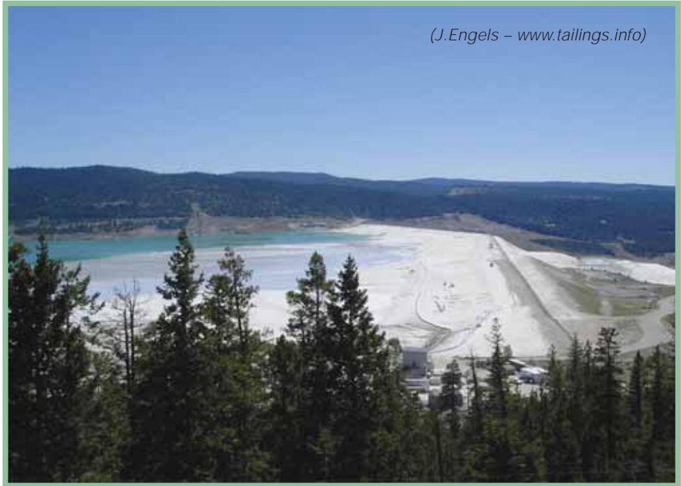
A tailings storage facility at the Highland Valley Mine in British Columbia.
