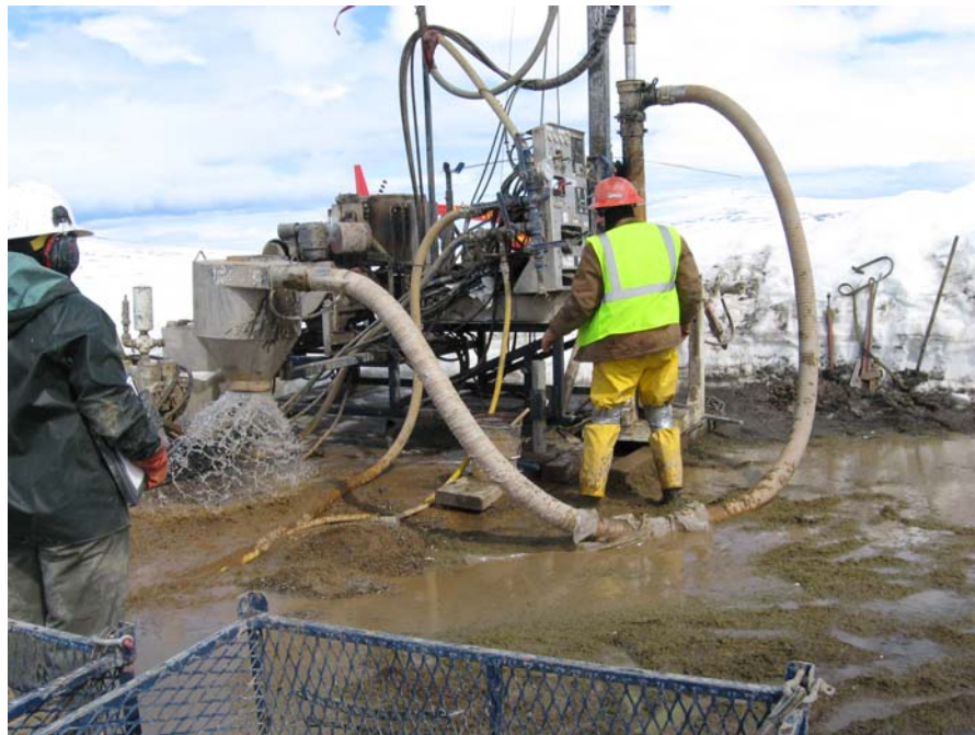
Figure 6. Groundwater monitoring well installation, drill rig number 8.
